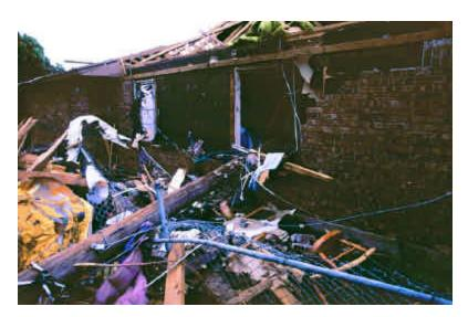
**Figure 30**. A power pole propelled through a window during the 3 May 1999 tornado in Del City, Oklahoma. It clearly did not tip over and through the window, since the top of the window frame remains intact (FEMA photograph by C. Doswell).
