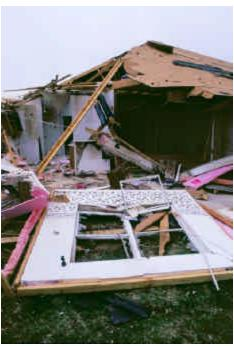
**Figure 43.** (Previous page) A frame home with little or no damage on its *front*, the side of the home facing the tornado. Note the damage to the home behind that in front, *farther* from the tornado (which has lost much of its roof), and the debris filling the space between homes in front. (Above) Damage to the *rear* of the home seen in the top photograph, caused by elements of the roof from the home across the street, behind it (FEMA photographs by C. Doswell).
