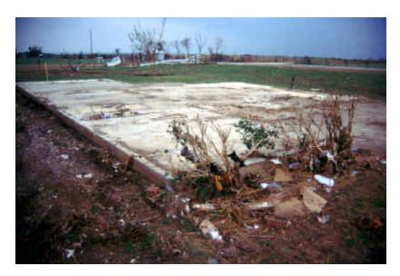
**Figure 27.** Empty slab left in the Double Creek Estates subdivision following the tornado of 27 May 1997 in Jarrell, Texas (Photograph © courtesy of T. Marshall, used by permission).
