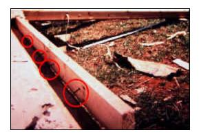
**Figure 12.** Straight-nailed bottom plate pulled out of the floor as the wall rotated. This was an inherently weak connection (circled).
