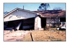
**Figure 21.** Inward failure of garage door led to outward failure of sidewall and collapse of the garage. Note little damage to remainder of home.
