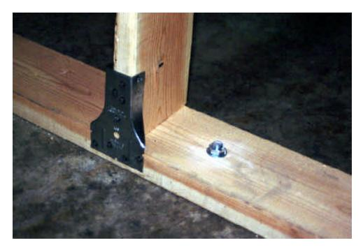
Figure A2.6. Example of a metal clip reinforcing the attachment of wall studs to the bottom plate. Note the bottom plate is bolted to the foundation with a nut and washer. [Photograph @ T. Marshall, used by permission]
