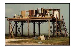
**Figure 18.** Wind damage to a home elevated on timber piles. Failure commonly occurs where the walls are attached to the floor.
