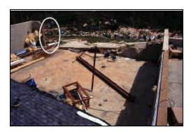
**Figure 13.** Exit door weakened the concrete wall foundation (circled). The foundation wall rotated and broke apart at the opposite corner. Steel rebar was used only at the wall corners. The house was pushed into the ravine in the background.
