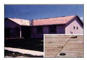
**Figure 26.** Poor installation of the roof covering on this home led to its complete removal. Staples were installed crooked and under-driven (inset photograph).
