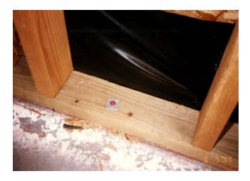
Figure A2.2. Attachment of bottom plate by shotpins. [Photograph © T. Marshall, used by permission]
