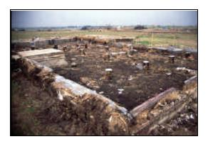
**Figure 10.** This home shifted and disintegrated from its wooden pier and concrete beam foundation. Floor joists were not attached to the piers.
