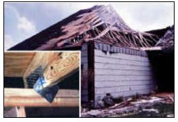
**Figure 24.** Toppled roof trusses due to a lack of lateral bracing. A metal bracket (inset photograph) along with proper wooden blocking between the trusses would have prevented rotation of the trusses.
