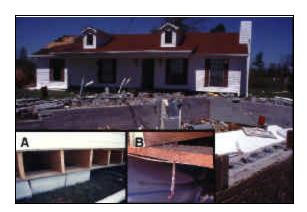
**Figure 15.** This home shifted off its foundation when the masonry foundation failed. Inset photograph A shows that the top row of masonry was attached with J-bolts as shown in inset photograph B. Note how little damage there was to the roof.
