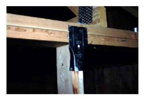
Figure A2.7. Example of metal clip reinforcing the attachment of the wall studs to the top plate. [Photograph @ T. Marshall, used by permission]
