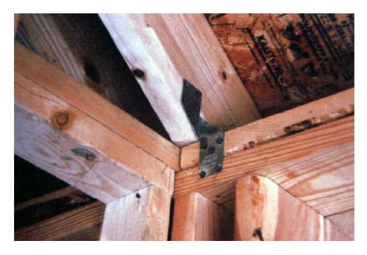
Figure A2.8. Example of a metal clip reinforcing the attachment of the roof trusses to the top plates. [Photograph @ T. Marshall, used by permission]
