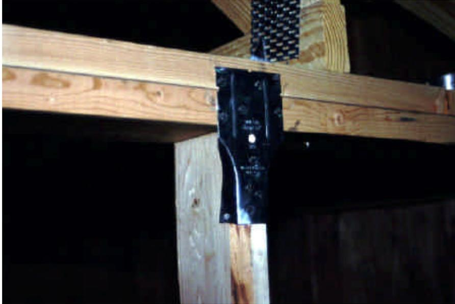
Figure A2.7. Example of metal clip reinforcing the attachment of the wall studs to the top plate.
