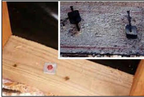
**Figure 7.** Shot pin with attached washer in the bottom plate. Inset photo shows aftermath of tornado where bottom plate broke around the fasteners.
