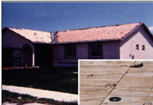
**Figure 26.** Poor installation of the roof covering on this home led to its complete removal. Staples were installed crooked and under-driven (inset photograph).
