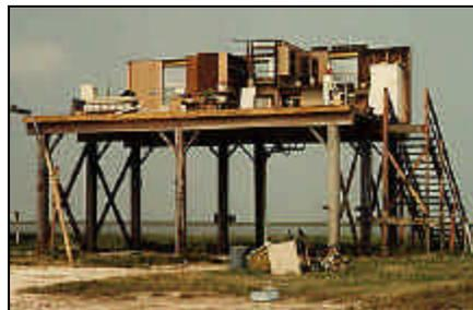
**Figure 18.** Wind damage to a home elevated on timber piles. Failure commonly occurs where the walls are attached to the floor.
