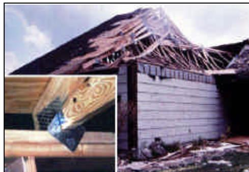
**Figure 24.** Toppled roof trusses due to a lack of lateral bracing. A metal bracket (inset photograph) along with proper wooden blocking between the trusses would have prevented rotation of the trusses.
