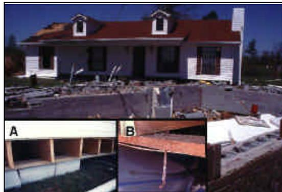
**Figure 15.** This home shifted off its foundation when the masonry foundation failed. Inset photograph A shows that the top row of masonry was attached with J-bolts as shown in inset photograph B. Note how little damage there was to the roof.
