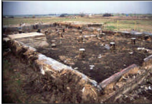
**Figure 10.** This home shifted and disintegrated from its wooden pier and concrete beam foundation. Floor joists were not attached to the piers.
