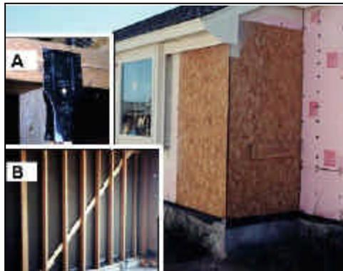
**Figure 19.** Installation of solid sheathing at wall corners helps stiffen the frame. Top plate clips as shown in inset photograph A and diagonal bracing as shown in inset photograph B also stiffen the frame.
