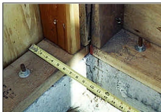
**Figure 2.** Properly bolted bottom plate. However, note the weak straight-nailed connection between the wall studs and bottom plates.
