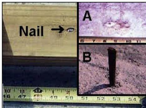
**Figure 8.** Cut nail in the perimeter bottom plate was a violation of the local building code. Inset photograph A shows scrape mark in the slab after wall slid off foundation. Inset photograph B is a cut nail left in the foundation after home was blown away.
