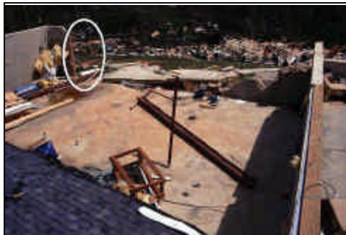
**Figure 13.** Exit door weakened the concrete wall foundation (circled). The foundation wall rotated and broke apart at the opposite corner. Steel rebar was used only at the wall corners. The house was pushed into the ravine in the background.
