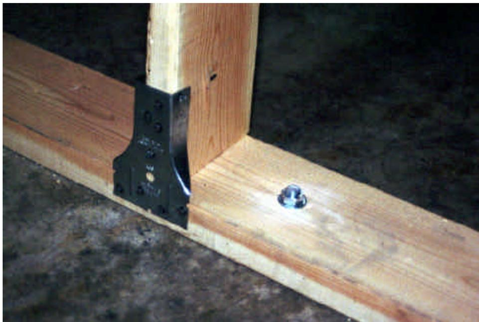
Figure A2.6. Example of a metal clip reinforcing the attachment of wall studs to the bottom plate. Note the bottom plate is bolted to the foundation with a nut and washer. [Photograph © T. Marshall, used by permission]
