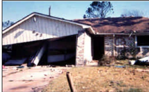
**Figure 21.** Inward failure of garage door led to outward failure of sidewall and collapse of the garage. Note little damage to remainder of home.
