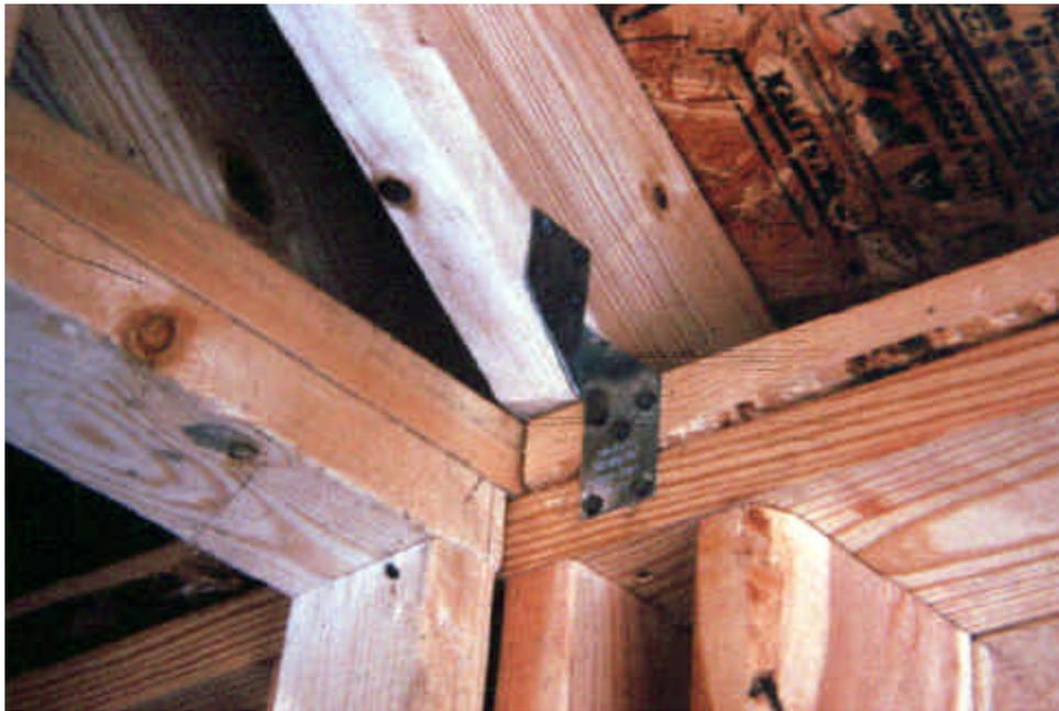
Figure A2.8. Example of a metal clip reinforcing the attachment of the roof trusses to the top plates.
