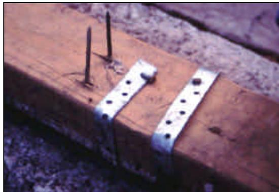
**Figure 6.** Metal straps held the bottom plate in place, however, failure occurred where the wall stud was straight-nailed through the bottom plate.
