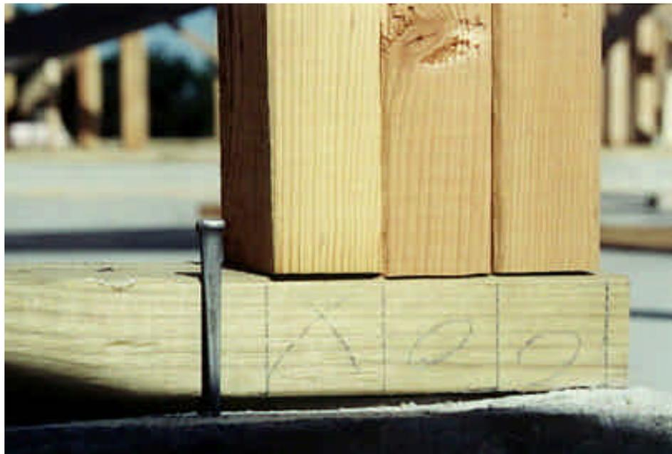
Figure A2.4. Cut nail, often powder-driven, used to attach bottom plate to foundation slab after the concrete has hardened. Note the relatively shallow penetration of the cut nail. Often, the impact of the nail shatters the concrete, leaving the nail essentially unattached to the concrete beneath the bottom plate. [Photograph © T. Marshall, used by permission]
