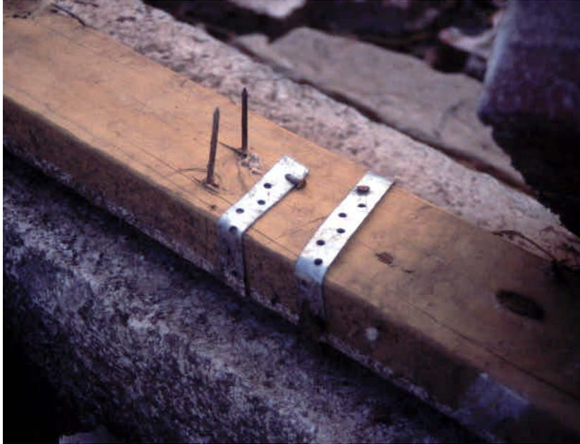
Figure A2.5. Bottom plate attached with strapping to the foundation, showing *straightnail* connection of wall studs to the bottom plate. The wall studs simply pulled out under lift forces, leaving the plate still attached to the foundation. [Photograph © T. Marshall, used by permission]
