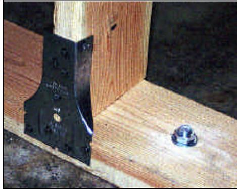
**Figure 5.** A metal clip connecting the wall stud to the bottom plate provides considerably more uplift resistance than conventional straight- or toe- nailing.
