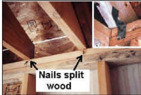
**Figure 23.** Nails driven through rafters and ceiling joists protruded through the top plate and split the wood. A better connection would have been to install metal clips as shown in the inset photograph that places the nails in shear (strong) instead of tension (weak).
